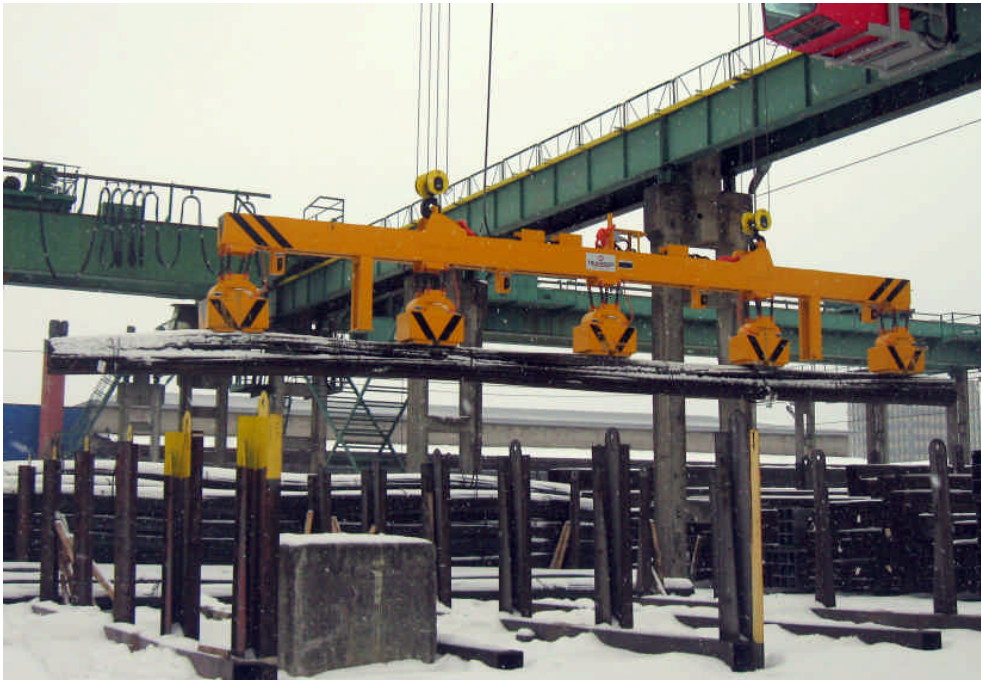
Figure 1: Handling of rebar bundles in the Baltic winter
